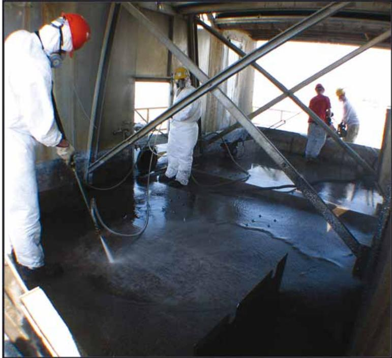
all dirt, debris, rust and corrosion leaving a clean profiled surface.
