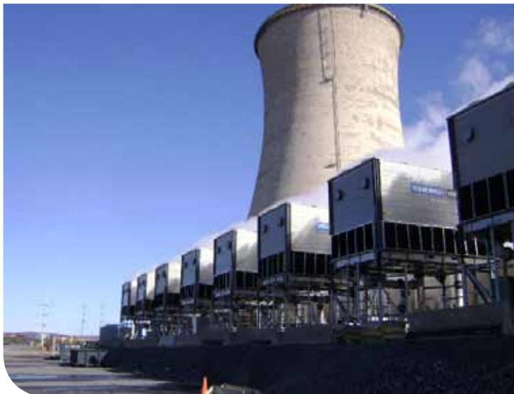
Temporary Cooling can also allow you to perform repairs to cooling equipment during regular operation hours, allowing you to concentrate on other issues during planned outages.
